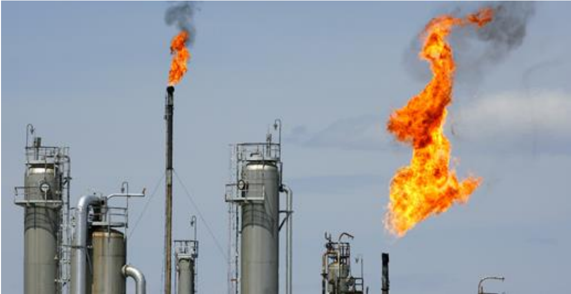
Figure 1.1 Flare stacks burn off gas at a natural gas processing plant [93]
