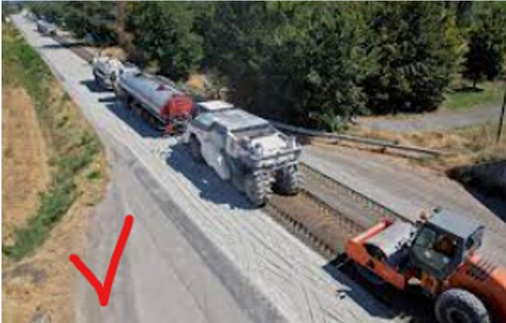
Joonis 4.4: Full-Depth Reclamation
