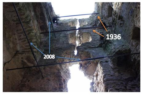
Figure 33. Steel anchors mounted into the SW tower to stabilize the wall movement
