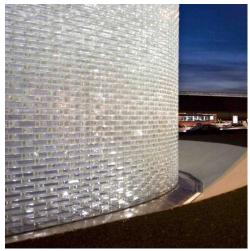
Figure 56. Glass masonry of Atocha
