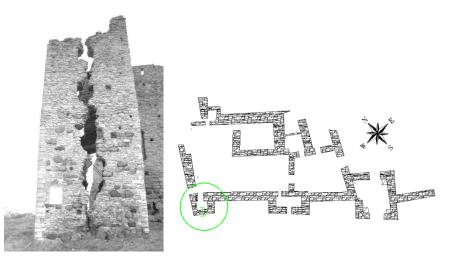
Figure 32. Extensive crack in the SW tower. Location of the tower
