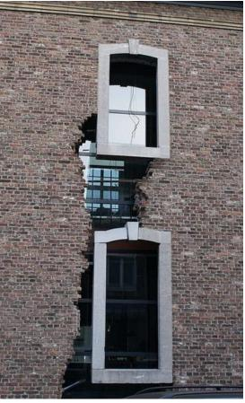
**Figure 26.** Multiple layers of float glass used to rebuild the ruined part of the mill [51]
