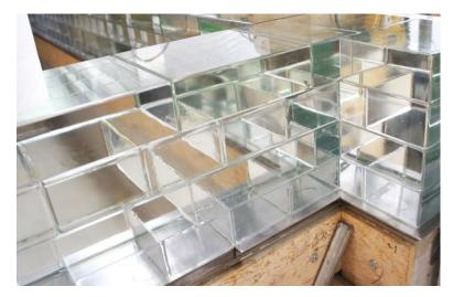
Figure 35. Glass block masonry system with transparent adhesive on horizontal surfaces and sealings on edge joints.
