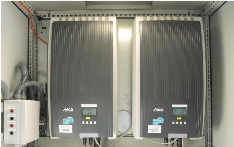
Figure 71 – Picture of the nanogrid's PV Inverters at the MCW.
