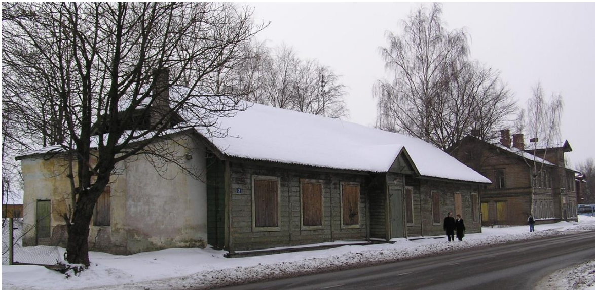
Photo 3.1-1 Vaksali 2e building before destruction [22]
