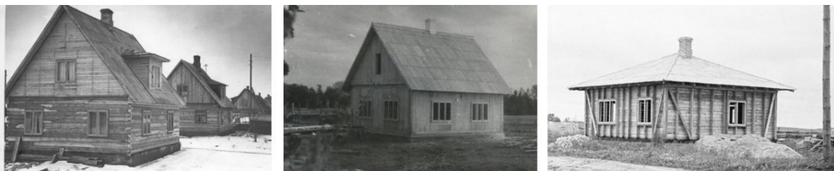
Figure 4.51 Examples of dwellings with timber structures (left to right: horizontal log (Võrumaa Muuseum, 1957), heavy timber frame with vertical logs (Valga Muuseum, 1957), light timber frame (Eesti Rahva Muuseum, 1962))
