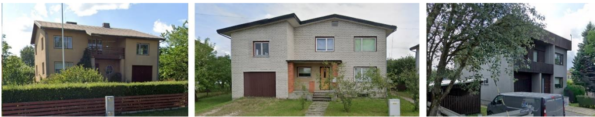
Figure 4.88 Examples of box houses with heated space above garages (left to right: Tartu mnt 44 (1984), Lepiku 17 (unknown year) in Karksi-Nuia; and Lõuna põik 10 (1982) in Väike-Maarja)
