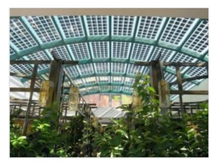
**Figure 8.** BIPV cladding systems (Topr-left: De Groot & Visser, Top- right: Sunpartner, Bottom: SELFA GE S.A) (Source: http://ashraemontreal.org)
