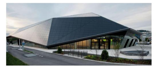
**Figure 5.** Umweltarena Spreitenbach (Switzerland 2012): an example of a 203% PlusEnergy building achieved by means of a customized 750 kWp full-roof BIPV skin consisting of c-Si panels with an antireflective glass (Architect: René Schmid Architekten; System provider : 3-S Photovoltaics, Meyer & Burger Group; Photo: Bruno Helbling)
