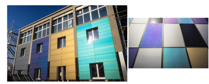
**Figure 13.** Basel, Switzerland, Kromatix<sup>™</sup> Glass: Grey, Blue, Blue Green and Gold, Surface Area: 159 sqm, Installed capacity: 24 kWp (Source: SwissInso).
