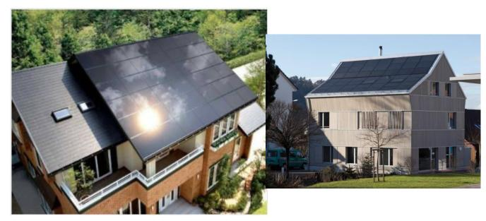
**Figure 6.** Fully covered in-roof installation, Left: (Source: NexPower Technology Corp.) Right: Einfamilienhaus in Glattfelden (Photo: Mirlo Urbano Architekten)
