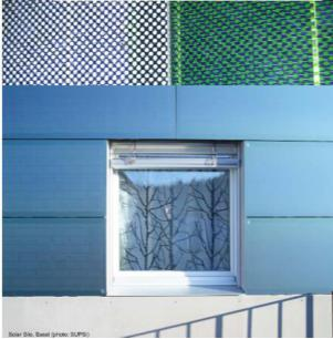
**Figure 15.** PV cells with ceramic digital printed front glass (Source: Left: SmartFlex Solarfacades), Right: Solar Silo (Basel)).
