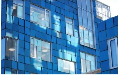
**Figure 12.** Location: Copenhagen, Denmark, Kromatix<sup>™</sup> Glass: Blue Green, Surface Area: 6,048 sqm, Installed capacity: 1,030 kWp (Source: SwissInso).
