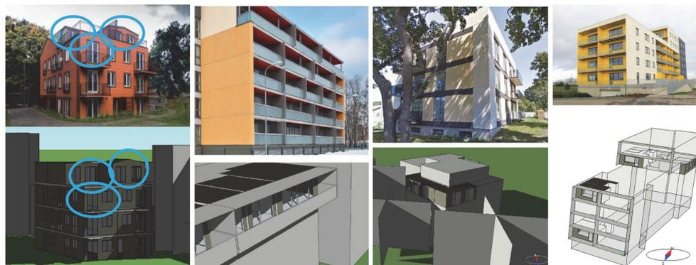
Figure 3. Example of modelled buildings with shading elements and selection of ‘critical’ rooms, which have highest potential to counter overheating. Photos (top) and simulation models (bottom).
