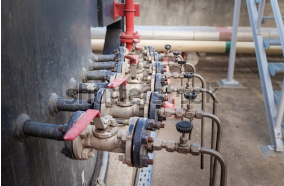
[6] Figure 10. different taps corresponding to different levels in the tank
