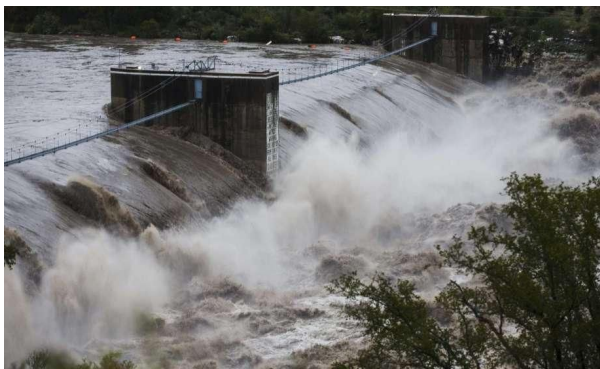
Figure 1.4.1H Flood over dam
