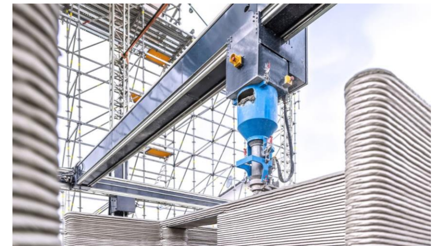
Joonis 12. Betooni printimine. Allikas: https://parametric-architecture.com/what-is-concrete-3d-printing/
