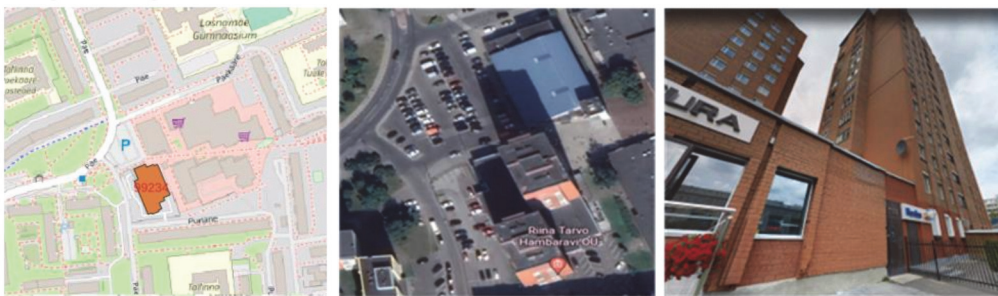
Case study 2: XY coordination based on Google earth: 59^{\circ}26'08''N24^{\circ}49'15''E Harju county, Tallinn, Lasnamäe district, Pae tn 68
