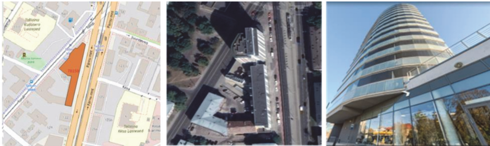
Case study 1: XY coordination based on Google earth: 59^{\circ}24'51''N24^{\circ}44'18''E Harju county, Tallinn, Kesklinna district, Pärnu mnt 110
