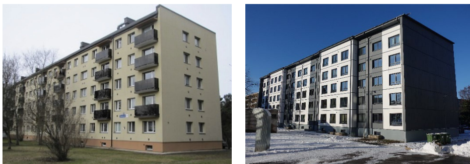
Figure 1.2 Complete energy renovation of apartment building with onsite renovation (left 2012) and offsite prefabricated renovation (right 2018).
