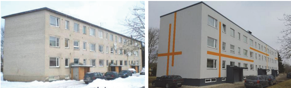
Fig. 1. Building 2.5 before (left) and after (right) energy refurbishment work has been carried out.
