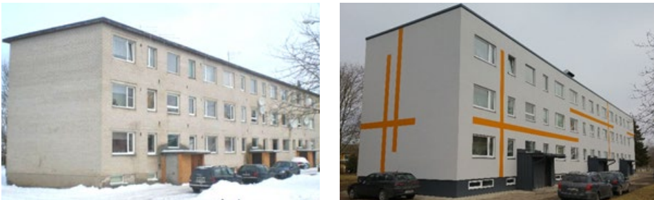
Figure 2.1 Studied apartment building before (left) and after (right) the deep energy renovation.
