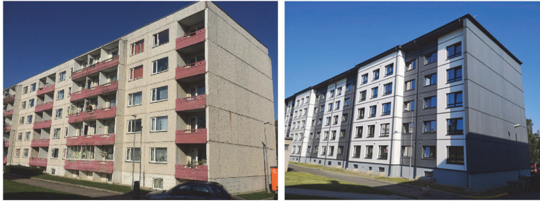
Fig. 1. View of the pilot building before (2015) (left) and after (right) the renovation (2018).
