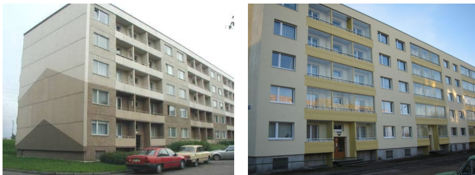
Figure 1.1 Development of renovation of apartment building over 15 years. In the beginning (left, 1993) only end-walls and roof were insulated, and the heating system was balanced. Later (right, 2008) the whole building envelope was insulated, windows were replaced, heating system was rebuilt. Mechanical ventilation with heat recovery is still missing today.
