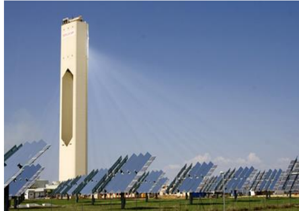
Figure 4.2: The Planta Solar 10 (PS10) is the world’s first commercial utility-scale solar power tower in Sanlúcar la Mayor, Spain [16].
