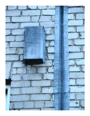
Figure 6 Breaches in building construction up to 0,5m have been covered with metal plates. Pärnu, Tallinn rd.1; photo by Tõnu Kütt
