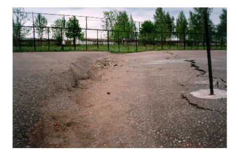
Figure 2 Subsided tennis court in town Kohtla-Järve, built without geotechnical engineering explorations. Underground mined area. Photo by Arvi Toomik
