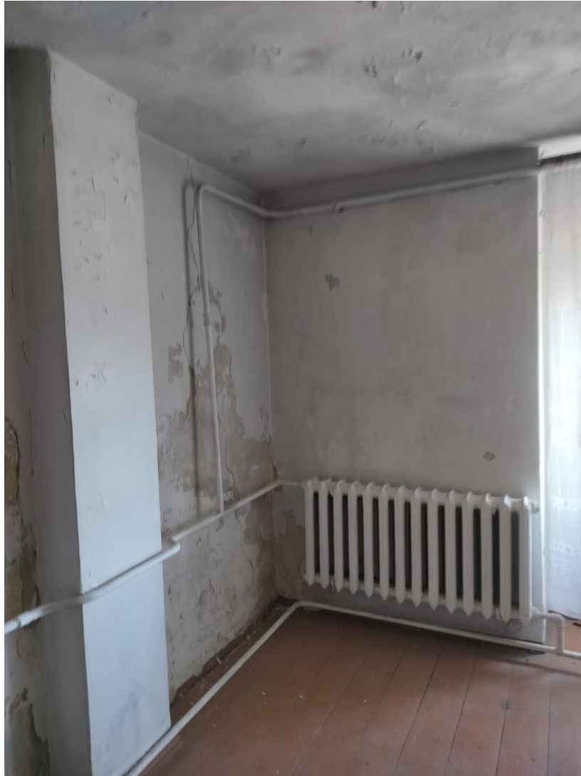
Figure 4. Decayed walls and legacy heating systems
