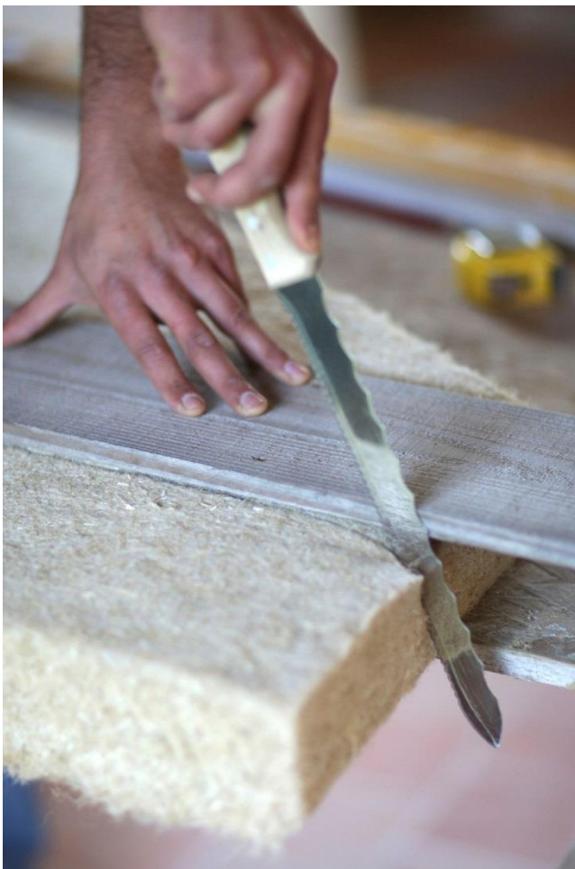
Figure 11. Cutting hemp fibre insulation [28]
