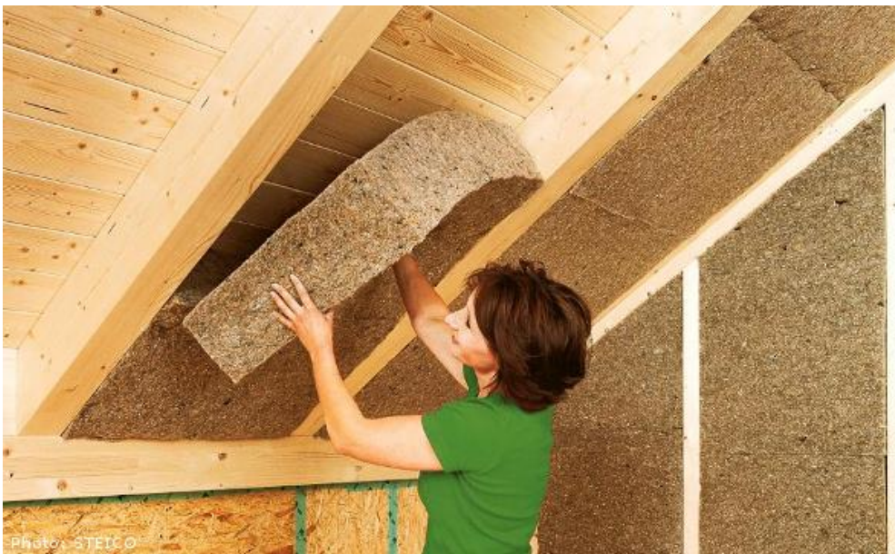
Figure 9. Woman installing hemp insulation [26]
