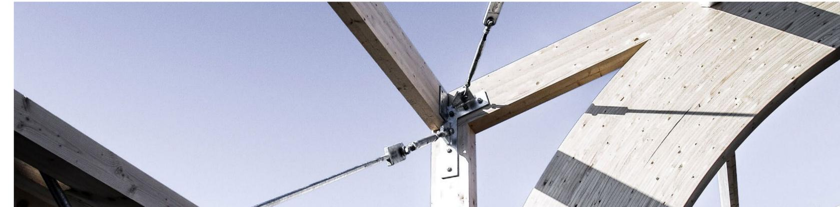
Figure 30. Construction joint done by *Límtré Vírnet* (*limtrevirnet.is*)
