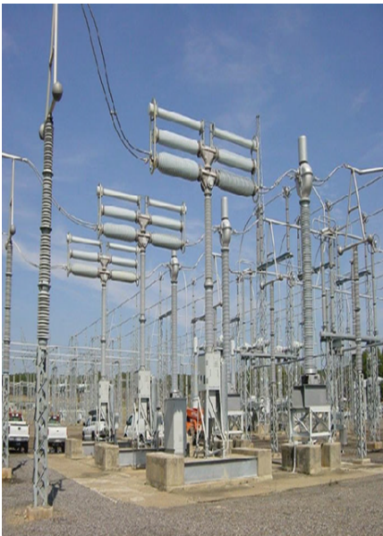
(c) 550 kV live-tank SF 6 gas circuit breaker
