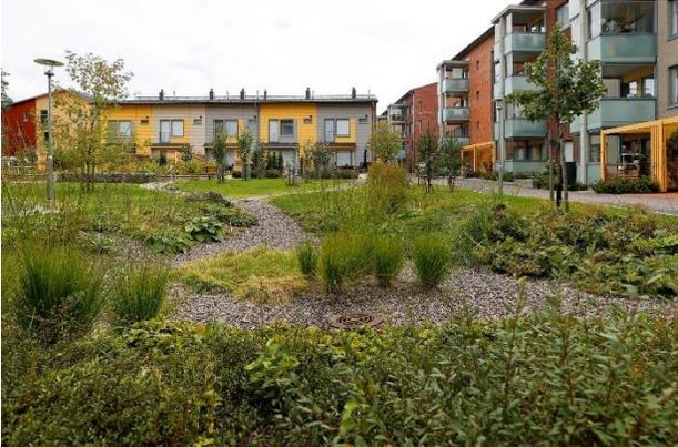
*Figure 33. Fannynkallio residential area of Helsinki where the topography was designed so that surface waters are directed to the rain gardens*
