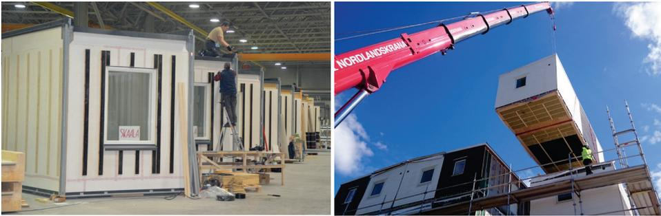
*Figure 1. Left: room module's manufacturing; right: on-site assembly. Photos by Harmet.*
