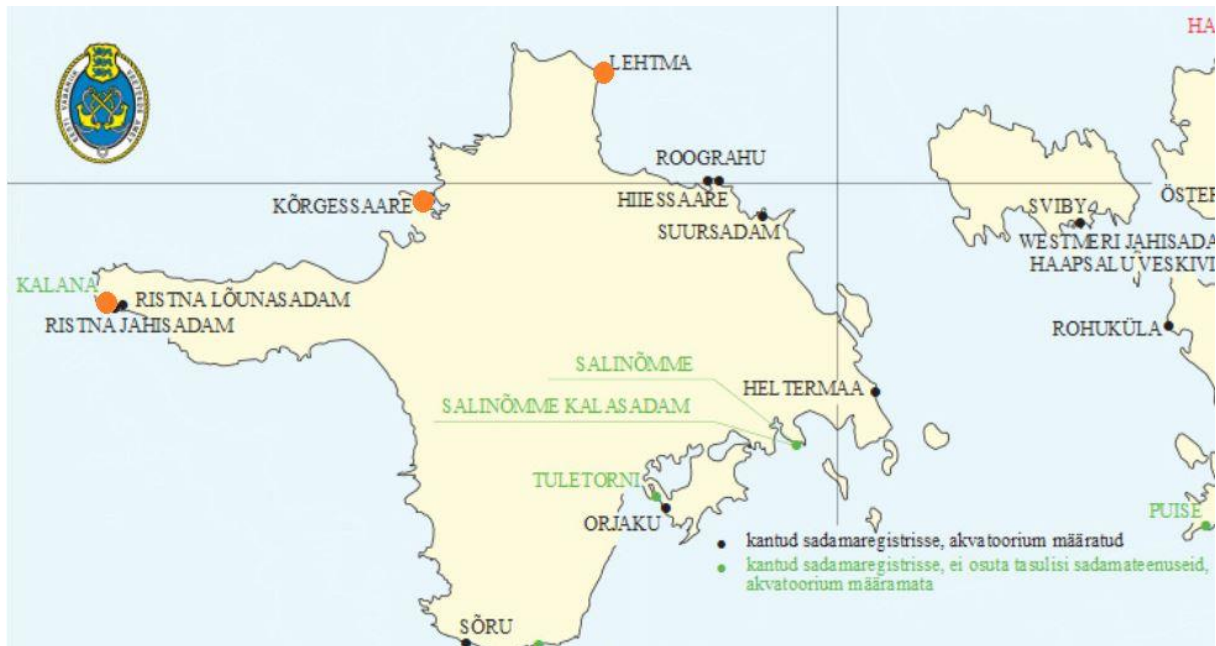
Figure 4. Three main ports Kalana, Kõrgessaare and Lehtma that will be used as onshore facilities for supporting maintenance [1]
