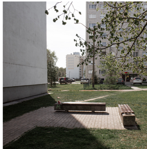
Figure 28: Typical existing seating area. Author's photo
