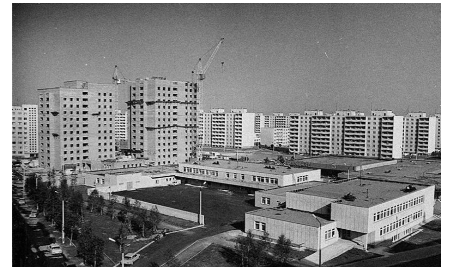
Figure 5: The construction of Lasnamäe
