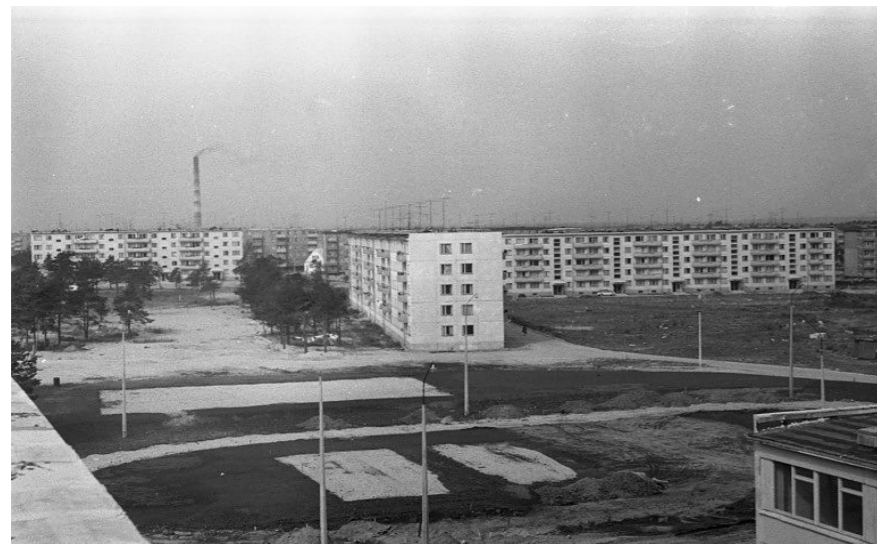
Figure 4: The construction of Mustamäe 5th district
