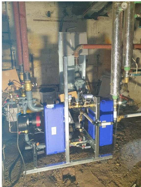
Figure 3.1. Picture of the new 2-stage heating substation at A36
