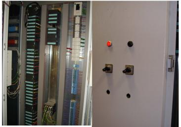
Fig. 4.12 Control terminal with a PLC and light and sound signaling.
