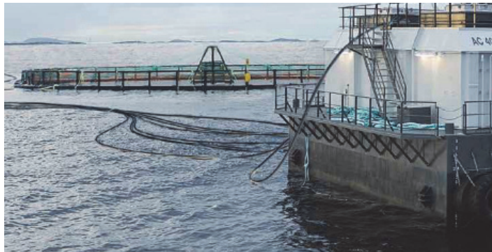
Figure 1.5. Cages with fish supply fed by the fish feeding barge [4].
