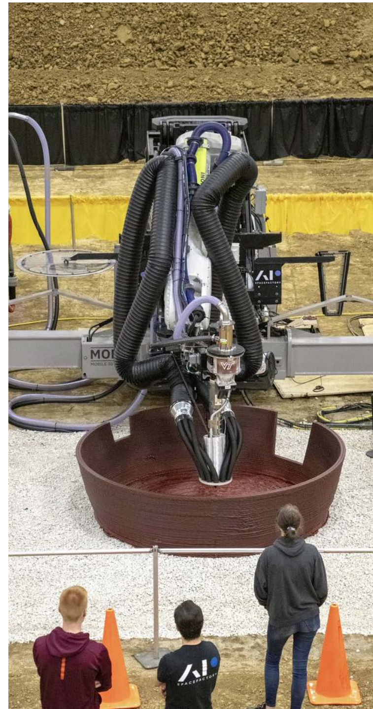
Figure 15. AI SpaceFactory prints a habitat for NASA's challenge (Staedter)
