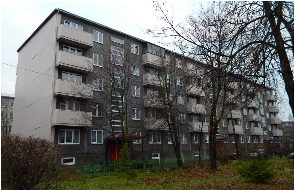
Figure 1.5. 1-464 series reinforced concrete apartment building in Tallinn, Estonia [8]
