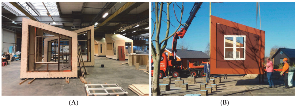
Figure 4. (A) Constructing the WikiHouse den Bosch. Source Tessa Peters and Rolf van Boxmeer; (B) Placing the WikiHouse Den Bosch. Source: Tessa Peters and Rolf van Boxmeer.
