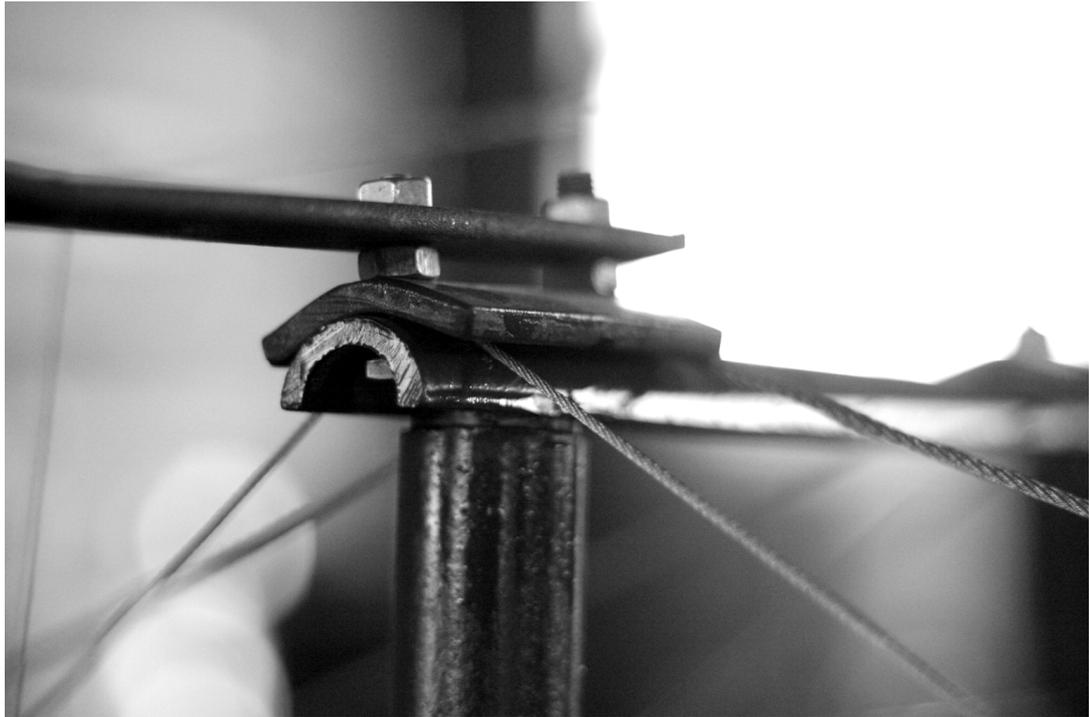
Figure 4.12 Anchoring the carrying cable and cable-stays at the top of the pylon.
