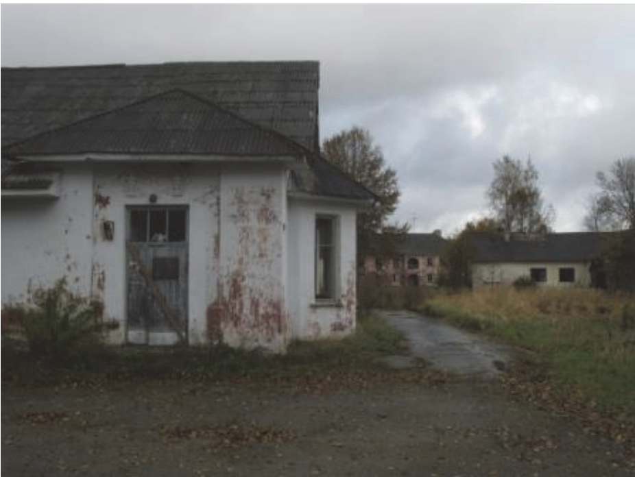
Figure 19. Viivikonna of Kohtla-Järve agglomeration, early-1950s, by Lengiproshacht. Photo taken in 2012. Source: EVM F 455.205.
