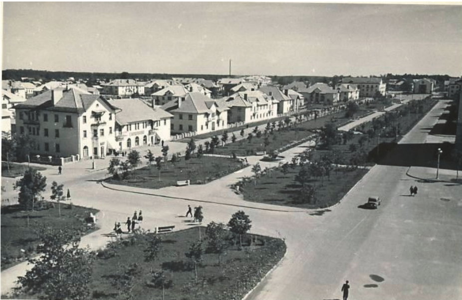
Figure 6. Stalinist centre of Kohtla-Järve, early 1950s by Lengorstroyprojekt (Jevsey Vitenberg, I. Pisareva, F. Kirzideli). Perspective view along the Victory Boulevard. Photo taken from crossing of the main axes in 1950s. Source: RM F 646.176.
