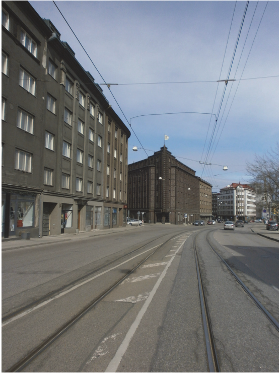
Fig. 1 Pärnu Road apartment buildings nearby Liberty Square in Tallinn from the late 1930s. Photo source: Siim Sultson
