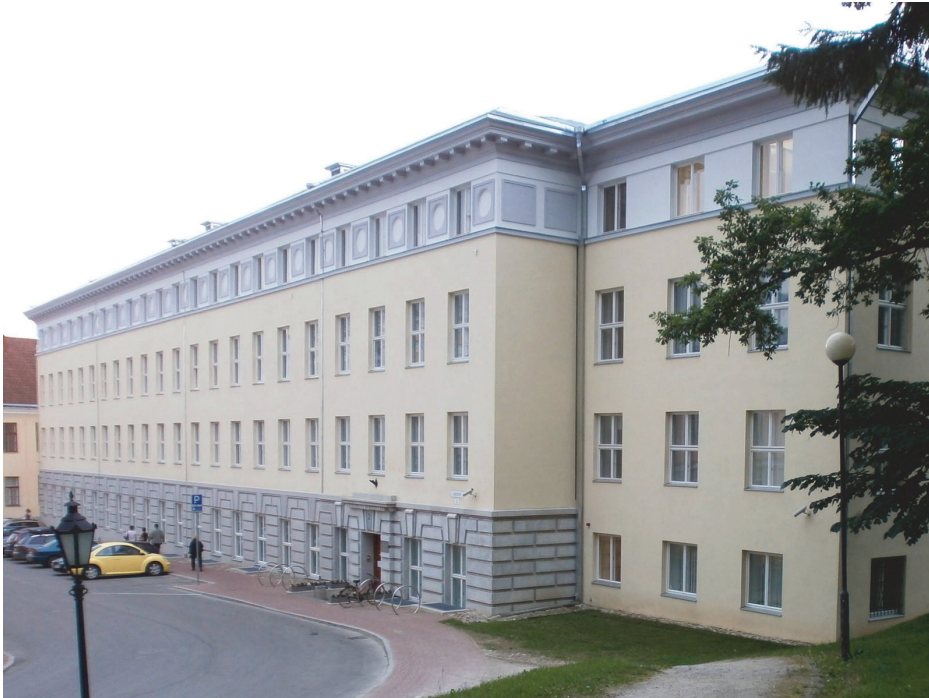
Figure 4. Institutes building of Tartu University, 1939–1942 by Harald Sultson. Source: Photograph by Siim Sultson 2013.
