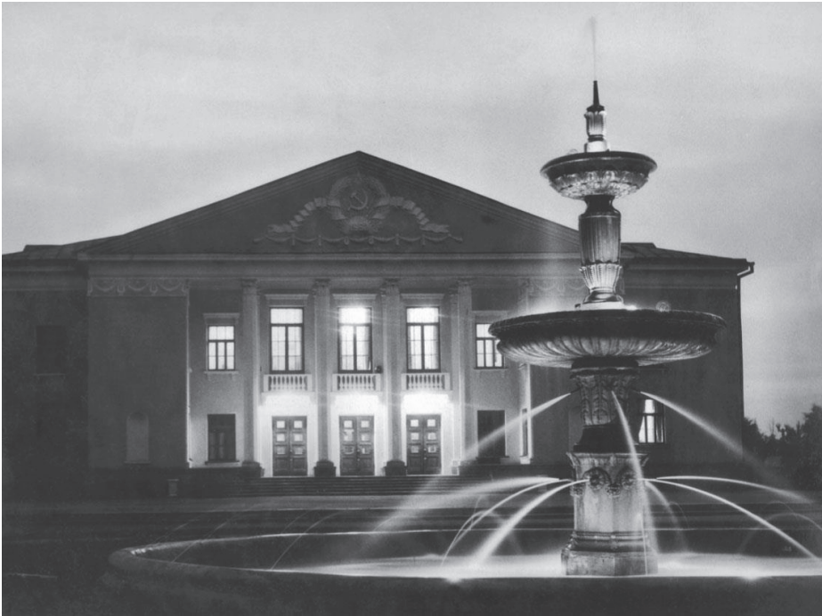
Figure 14. The Palace of Culture in Kohtla-Järve centre (Järve), early-1950s by Lengorstroyprojekt. Photo taken in 1952. Source: Eesti Entsüklopeedia, 2017.
