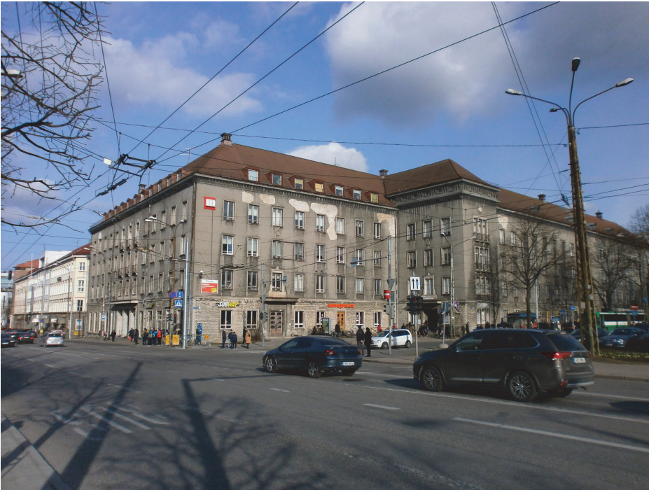
Figure 7. Estonia Boulevard administrative buildings opposite Estonia Theatre in Tallinn from the turn of 1940s and 1950s. City space of the Cultural Centre in Tallinn by Harald Arman, the front building, 1948–1953 by Enn Kaar. Source: Photograph by Siim Sultson 2017.
