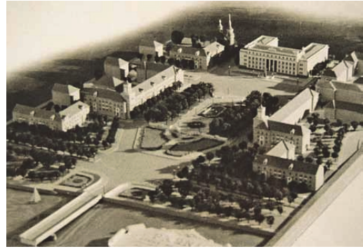
Fig. 6. Pärnu oblast centre by Harald Arman, 1952–1955. On the site of the demolished Old Town and ruins of the Teutonic Castle (EAM 3.1.323)
