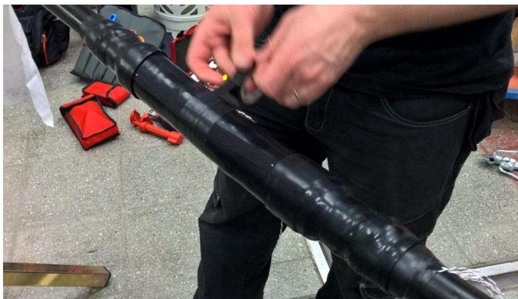
Figure 4.5. Finished cold shrink joint.
