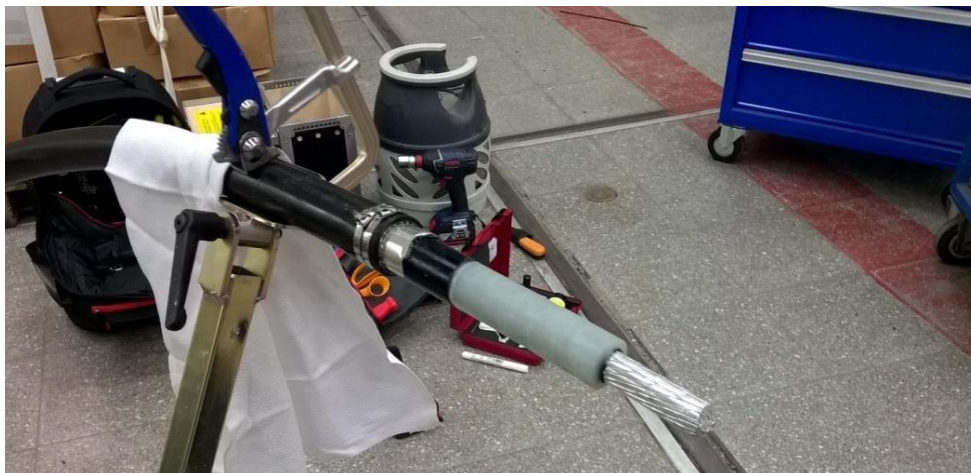
Figure 4.1. Cable end after preparing. It already includes an aluminium detail that connects to the aluminium foil under the cable jacket.
