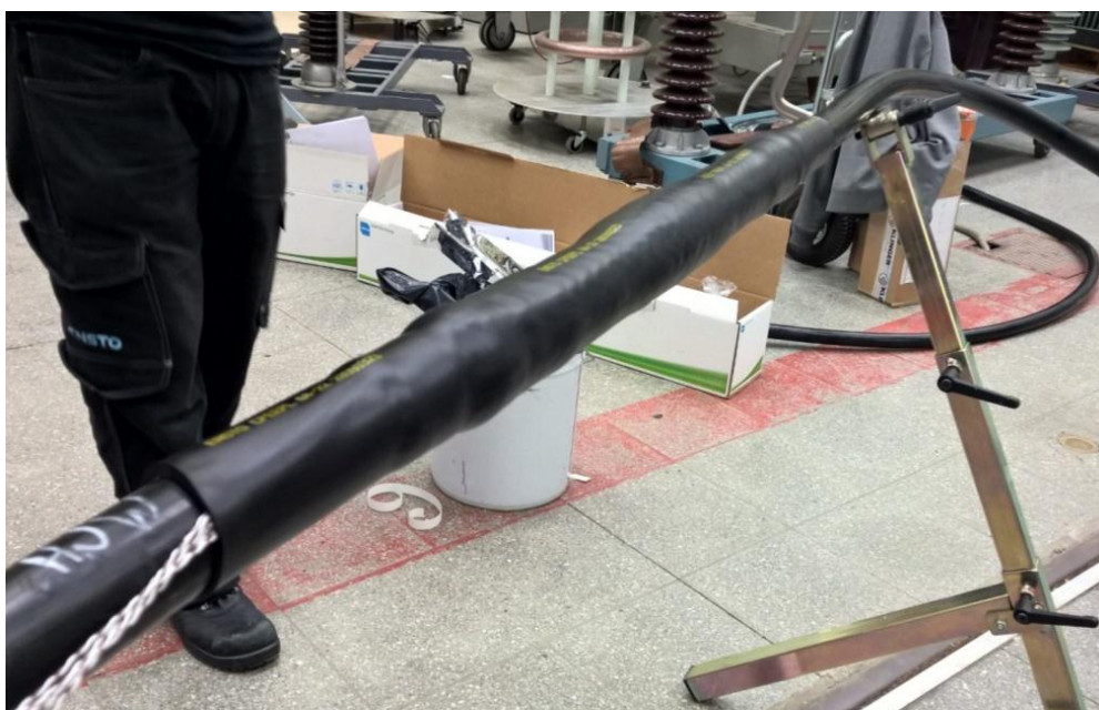
Figure 4.9. The finished heat shrink joint.
