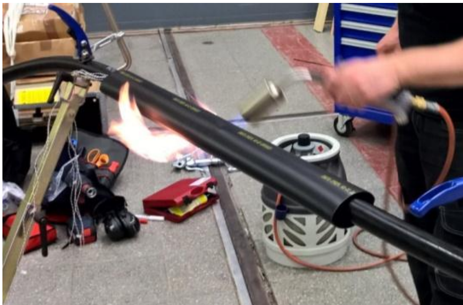
Figure 4.8. The final layer being applied onto the joint.
