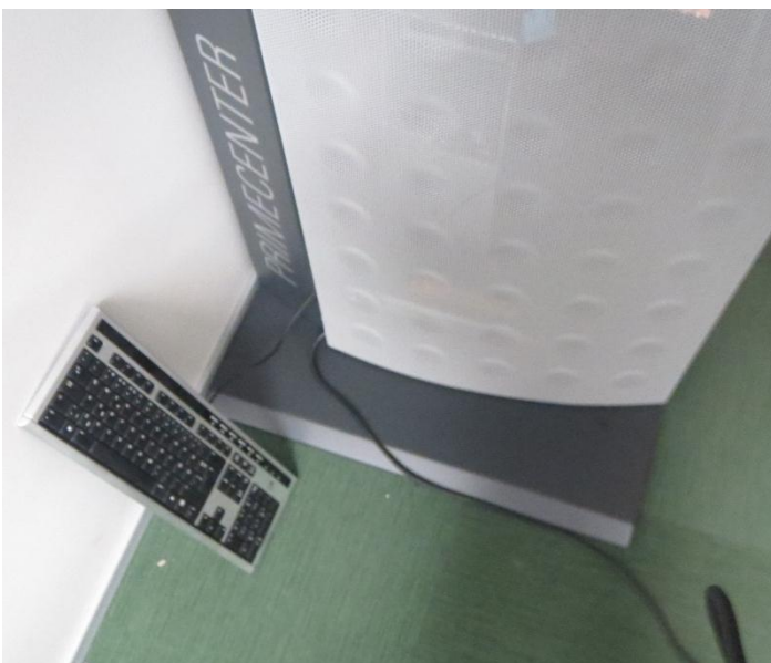
Figure [9] Protruding footprint of Fujitsu rack cabinet
