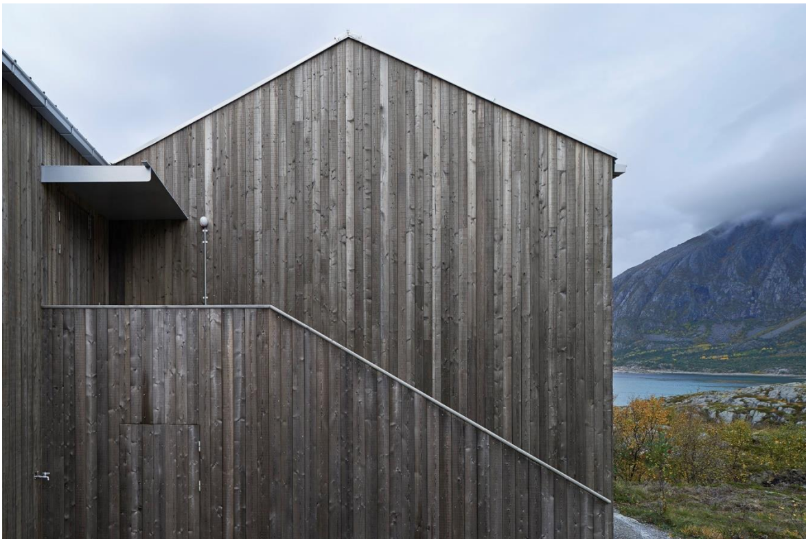
Figure 2.2. Weathered wooden facade (Lindman, 2014)
