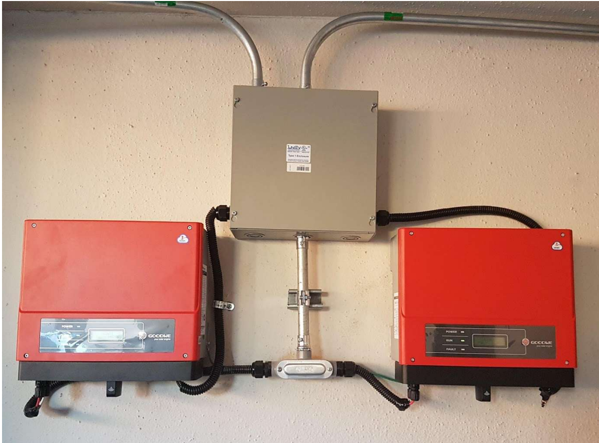
Picture of the two solar inverters
