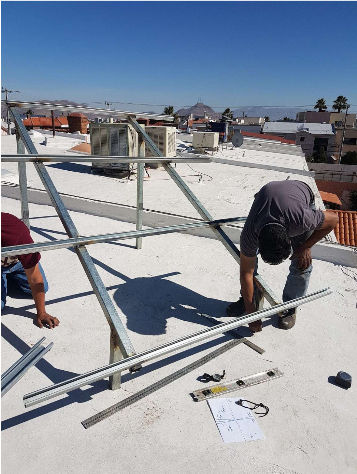
Process with installation, note the compass used to calculate the magnetic south.
