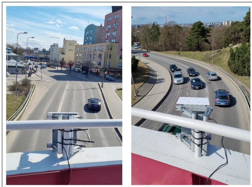
Figure 36. Mounted hardware on both sides of the bridge
