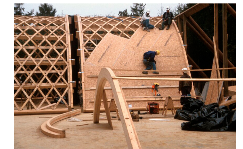
Figure 37. Filmwell Woodland Enterprise Centres modular timber gridshell. Source: Atelier Ten
