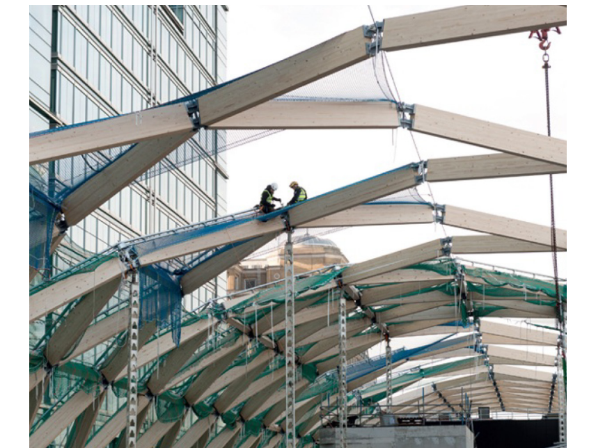
Figure 42. Construction in progress. Source: Foster + Partners
