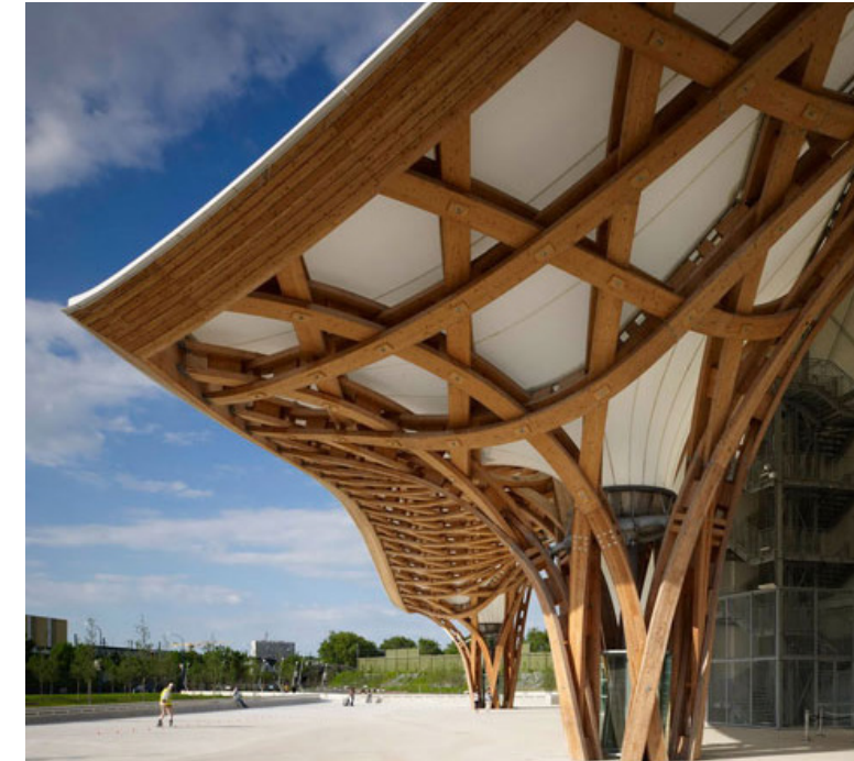
Figure 33. Hexagonal grid roof of the Centre Pompidou – Metz. Source: Shigeru Ban Architects
