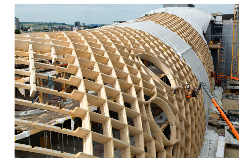
Figure 47. Construction in progress Source: Archdaily
