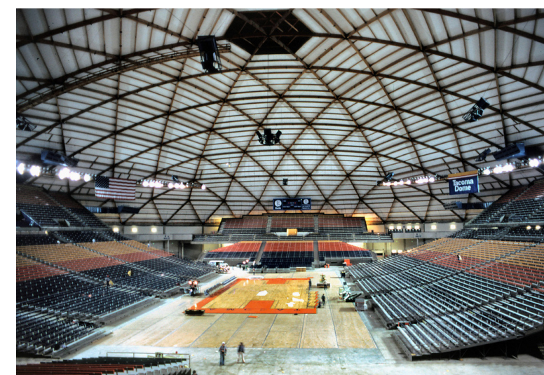
Figure 34. Triangular grid of the Tacoma cupola. Source: SPS+ Architects
