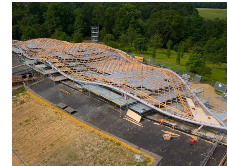
Figure 31. Construction in progress. Source: Glenn Howells Architects
