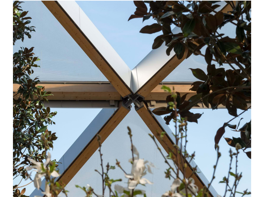
Figure 41. Nodal connection. Source: Foster + Partners
