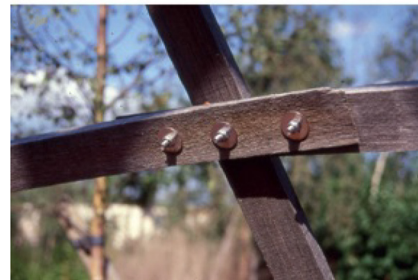
Figure 20. Earth Centre timber gridshells. Source: Chilton, J.C., Tang, G. (2016)
