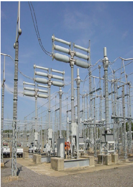
(c) 550 kV live-tank SF 6 gas circuit breaker
