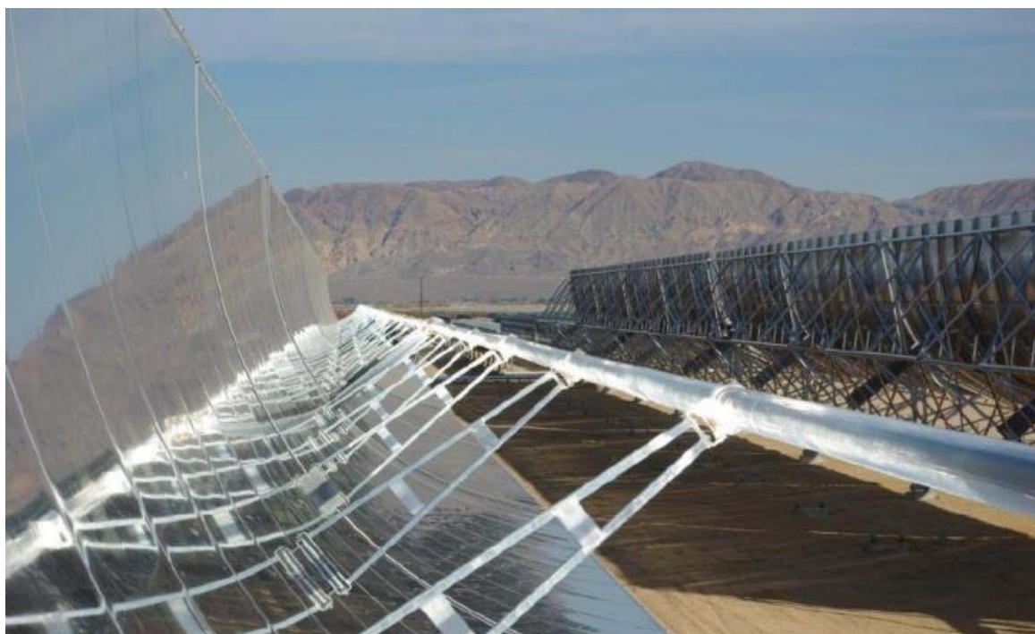
Figure 11. Skytrough SCHOTT PTR80. (34)
