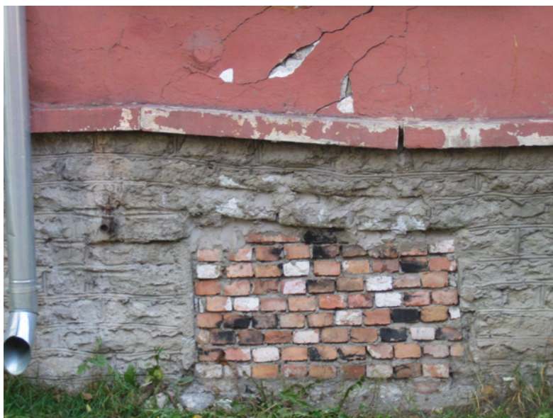
Effects of differential settlement
