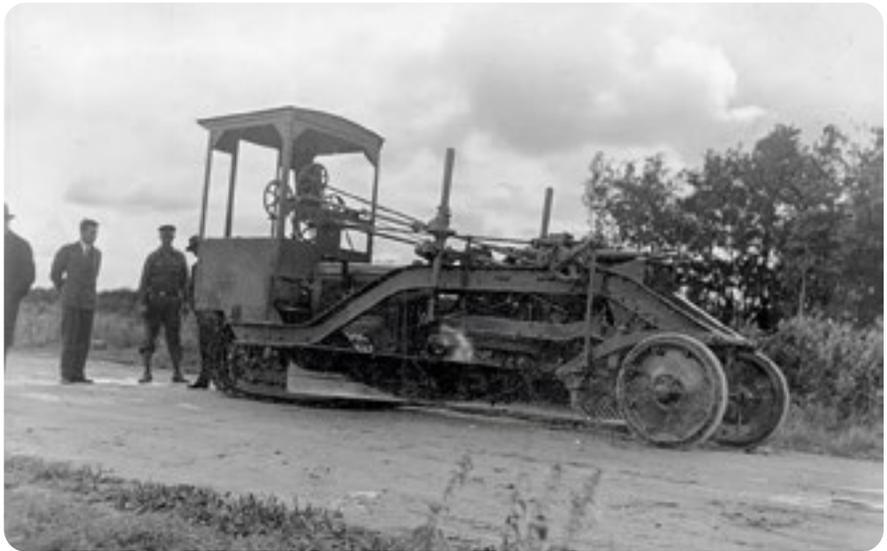
Court tested the machine on the Tallinn-Haapsalu road where the road was covered with crushed granite, which was unsuitable for the graders already in use. The machine was approved, and Harju County Court made the Ministry of Roads the proposal to buy the grader from Franz Krull, which was done in 1932.<sup>32</sup>
