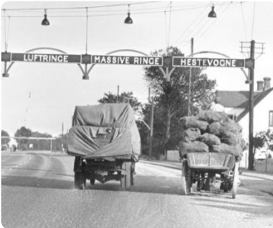
*In 1926, an experimental facility was established on Roskildevej, the central road to Copenhagen, which was prepared for three types of transport: horse-drawn carriages, carriages with solid tyres and vehicles with air tyres. The experiment readily revealed how much a road would be worn after the passage of increasingly more vehicles. (Glostrup Lokalhistoriske Arkiv)*
