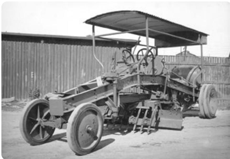
*A Talkoo-motor grader built by the Ahjo company in 1933. The eventual machine was almost identical to the ones built by Tiekone company. (Mobilia, Väyläviraston kokoelma, Nyblin)*
