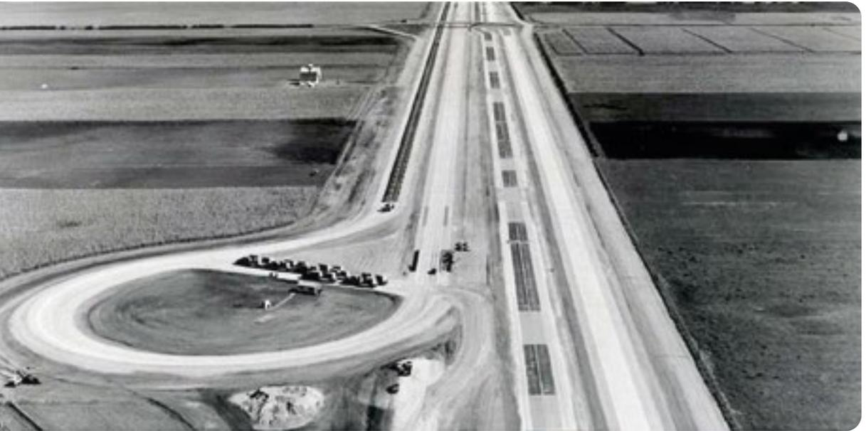
*In the United States, outside Ottawa, Illinois, the construction of six test tracks in 1956 started to shed new light on road structures. The tracks were supposed to amount to an extensive network of highways between the states. Today, remaining parts of the lanes form part of Interstate 80. (Washington State Department of Transportation)*
