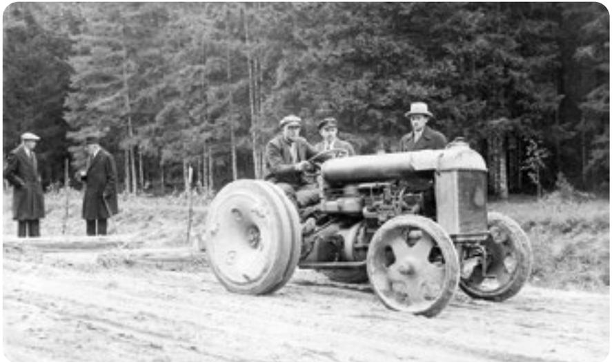
ment found that the grader ploughs were completely unsuitable for snow clearing. Fresh snow carried the plough, which was equipped with a sleigh, but the front wheels of the grader sank into the snow and moving forward became difficult. Only the blade of the grader cleared the road in this case whilst the snow plough simply slid across the snow.<sup>27</sup> Attempts to use road graders in snow clearing nevertheless continued from 1928.
