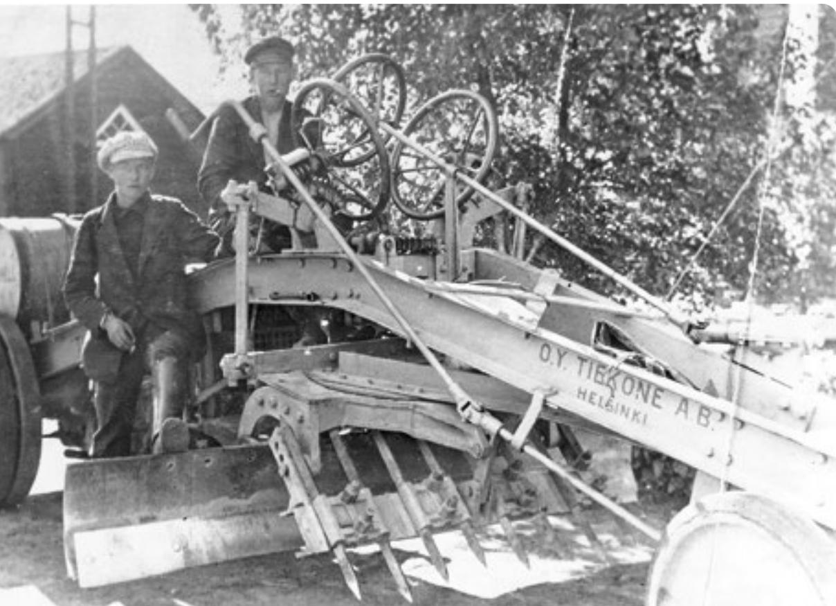
*An early Tiekarhu in Ostrobothnia. Tiekarhu no:3, still equipped with tilting front-wheels, was given over to the Vaasa Road and Water District.*
