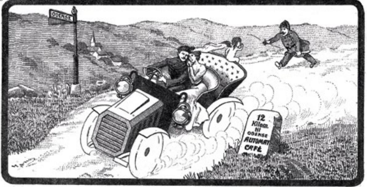
*Advertising for early cars showcased the problems that passenger cars caused for Denmark's roads. Their fast rubber tyres sucked up the sand, such that new-and-improved roads literally disappeared in a cloud of dust. The first task of road engineers was thus to secure the surface of the roads.*
