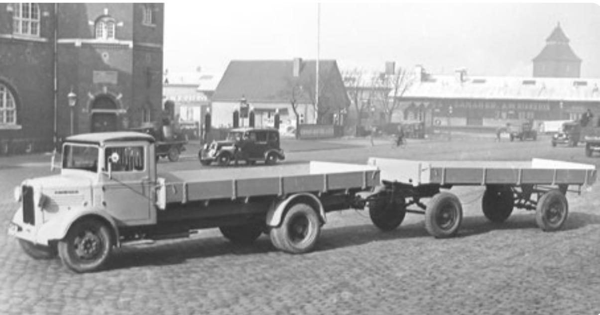
*Using a trailer was a method of enabling a truck to pull nearly twice as much weight as it can on its own, and once trucks were installed with equipment using compressed air, trailers could be braked. The number of trailers in Denmark first exceeded 1,000 in the early 1930s. (Danish Veteran Car Club)*
