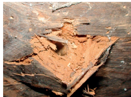
Figure 4: Wooden floor on roundwood beams (left) damaged by rot and insects (right).
