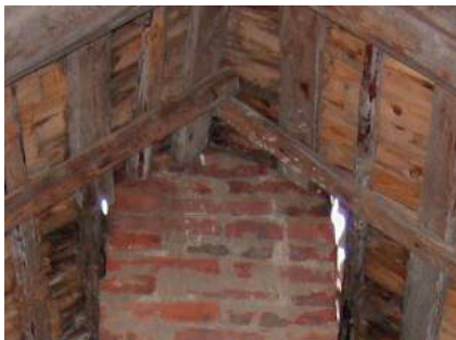
Figure 11: Typical leaks: around the chimney (left) and due to excessively old roof covering (right).
