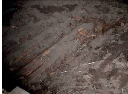
Figure 10: Fire risk in the attic (left). Rot damage to wooden ceiling details insulated with soil.
