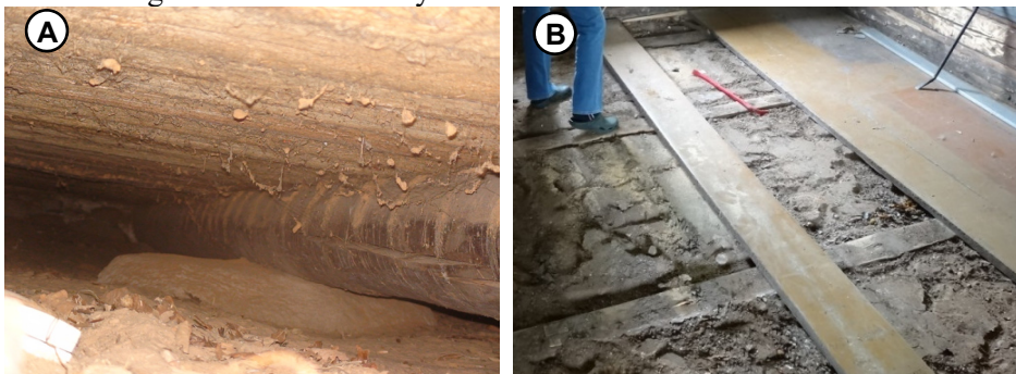
Figure 4.3. Wooden floor on roundwood beams (A). Floor beams inside damp soil (sand) (B).
