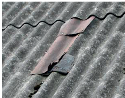
Figure 11: Typical leaks: around the chimney (left) and due to excessively old roof covering (right).
