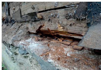
Figure 7: The bitumen paper behind the external boarding that should stop the rain load on the log is broken and has clogged the air layer behind the boarding (right). Missing waterproofing between the foundation and the log and the mortar above the log result in rot damage to the lower log (right).
