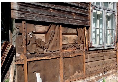
Figure 7: The bitumen paper behind the external boarding that should stop the rain load on the log is broken and has clogged the air layer behind the boarding (right). Missing waterproofing between the foundation and the log and the mortar above the log result in rot damage to the lower log (right).
