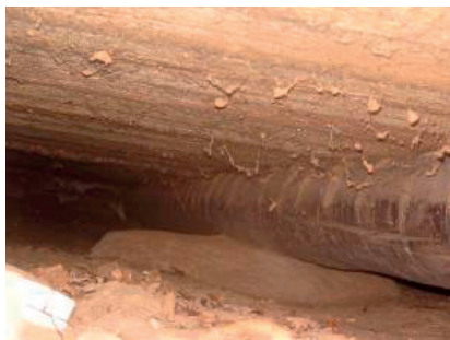
Figure 4: Wooden floor on roundwood beams (left) damaged by rot and insects (right).
