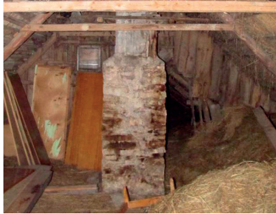
Figure 10: Fire risk in the attic (left). Rot damage to wooden ceiling details insulated with soil.
