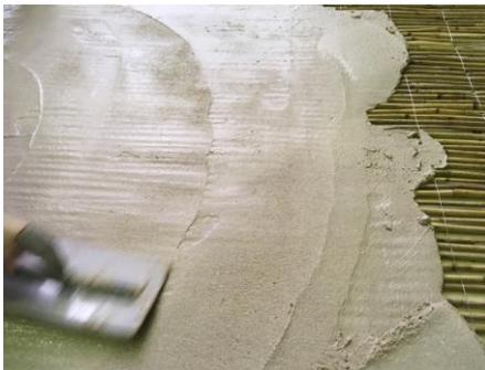
a) Application of the first layer of lime plaster using a trowel.
