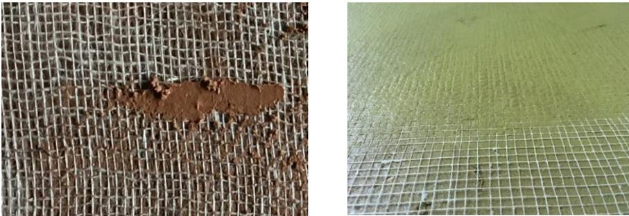
Figure 3-4. Application of reinforcement mesh into the clay plaster system: Left – Jute mesh; Right – Flax mesh embedded in the plaster.
