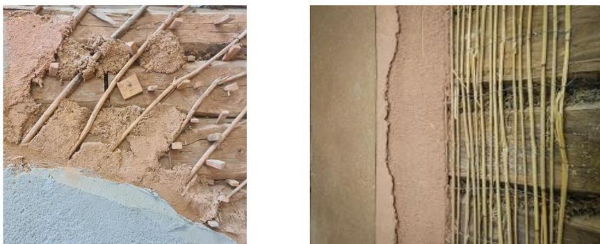
*Figure 3-2. Examples of plaster support fixed on horizontal-log construction for the mechanical fixation of plaster: Left – Plaster applied on wooden lath and sticks. Right – Reed mat fixed to a log wall by using staples.*
