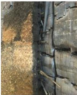
a) Clay plaster after the detachment of the outer plaster layers on timber.
