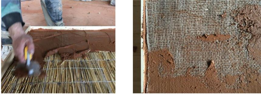
*Figure 5-19. Plasterwork carried out in all test programs: Left – Application of a first plaster layer on a reed board; Right – Jute mesh applied on a plaster layer.*
