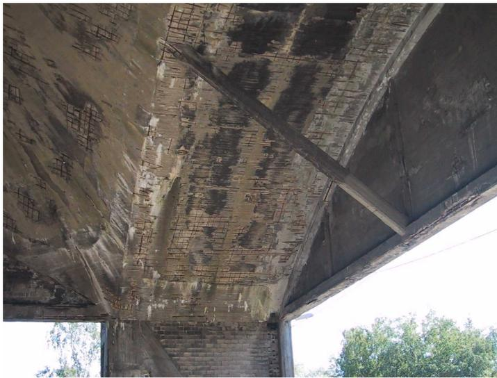
Figure 5.3 Reinforced concrete angle braces used to take wind loads
