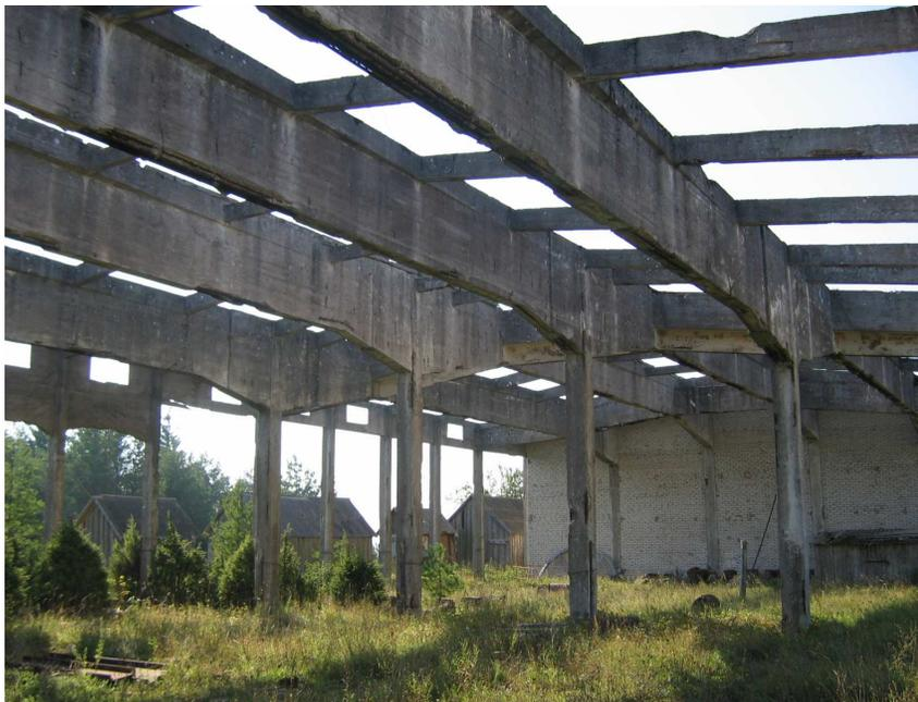
Figure 5.11 Damages of the hangar frame
