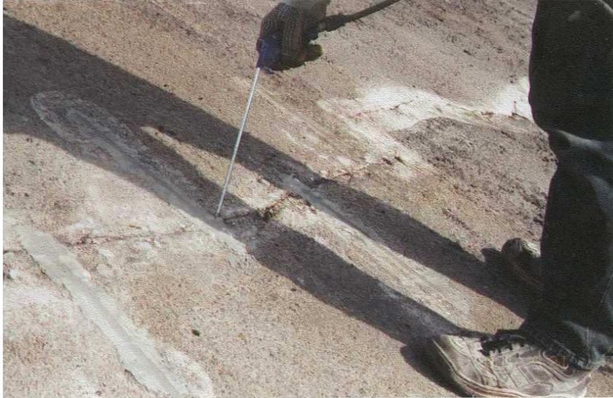
Figure 7.9 Cleaning of cracks in the shell before injection of epoxy resin
