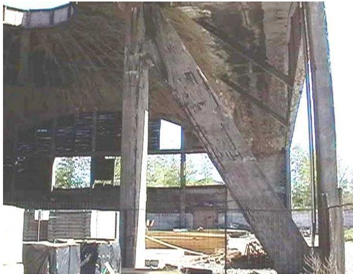
Figure 5.2 Reinforced concrete columns and angle braces
