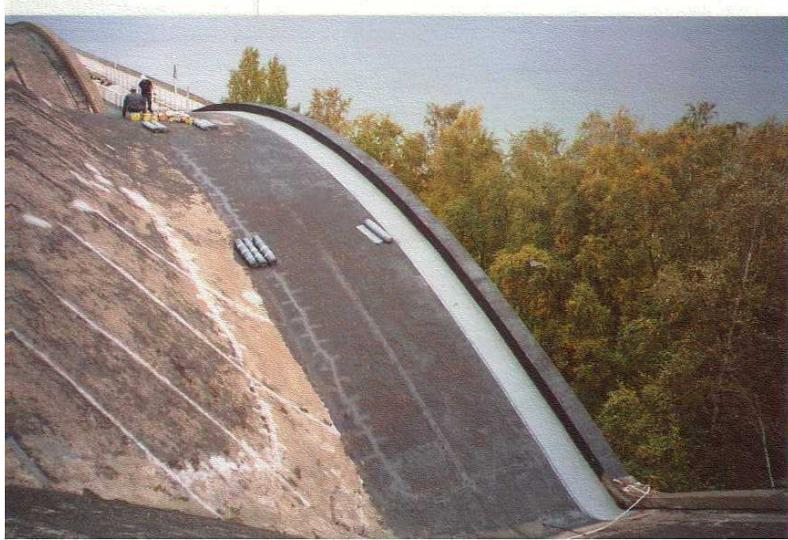
Figure 7.13 Installation of roof cover
