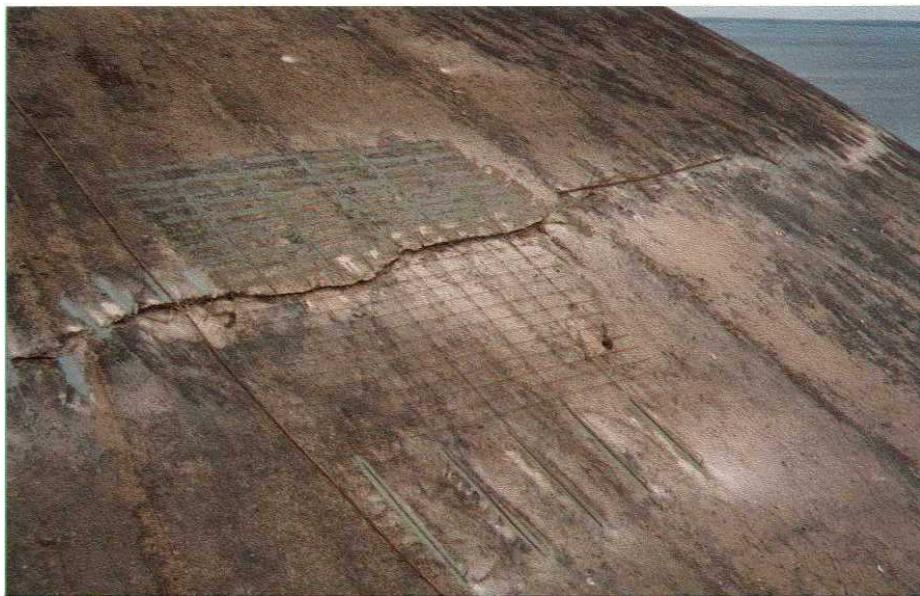
Figure 7.3 Reinforcement bars-anchor fixed to the canal by glue mixture in the deformed spherical shell area
