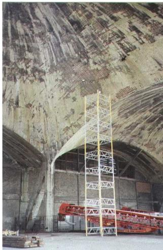
Figure 7.1 Supports to the deformed area of the spherical shell
