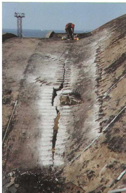
Figure 7.5 Reinforcement of the interface area of the spherical and cylindrical shell
