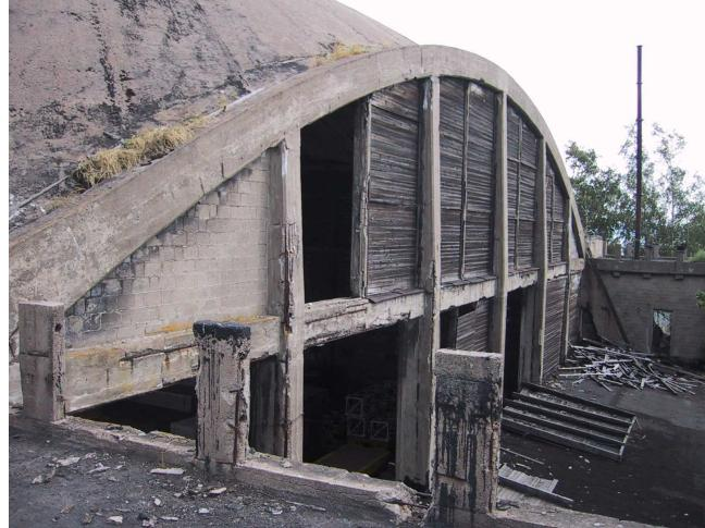
Figure 5.4 Edge element of the shells and girder covered by timber slatings
