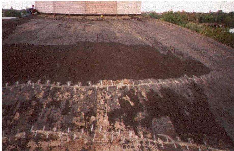
Figure 7.11 Cracks stitched and injected by epoxyl resin
