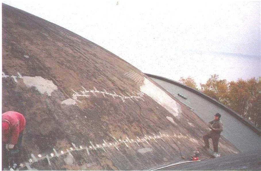
Figure 7.4 Reinforced and monolithic area of deformation in the spherical shell
