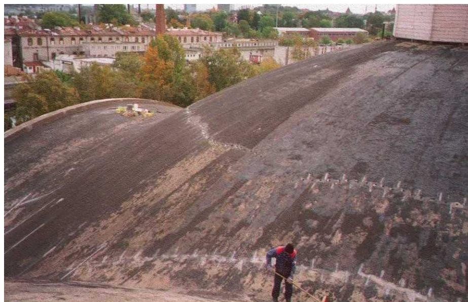
Figure 7.12 Cleaning of shell cover from old roof coverage
