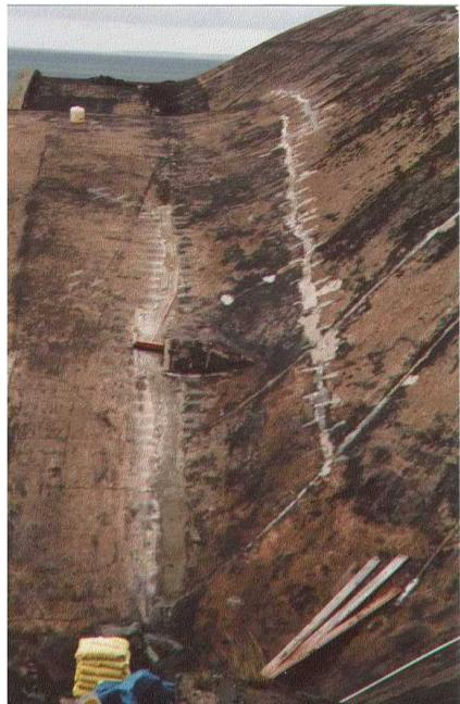
Figure 7.6 Monolithicizing of the interface of the spherical and cylindrical shell
