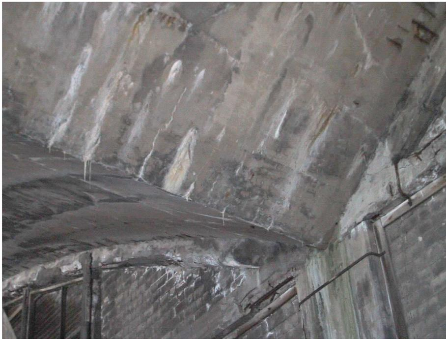
Figure 5.19 Stalactides suspending from the lower shell surface
