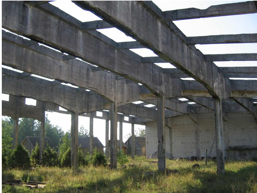
Figure 5.11 Damages of the hangar frame
