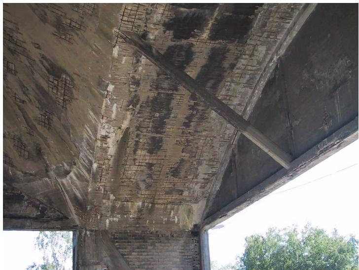
Figure 5.3 Reinforced concrete angle braces used to take wind loads
