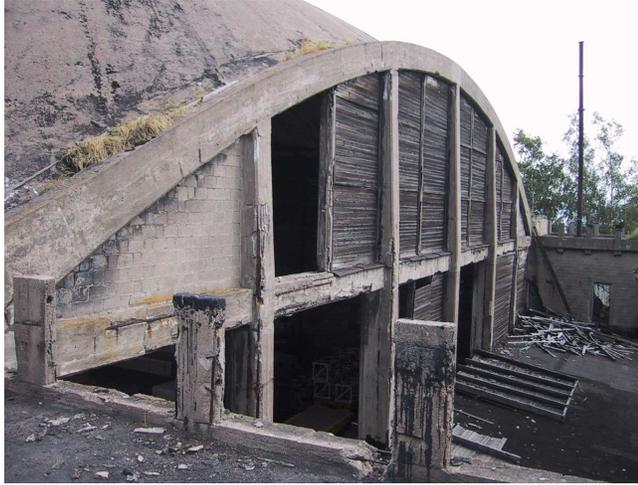
Figure 5.4 Edge element of the shells and girder covered by timber slatings
