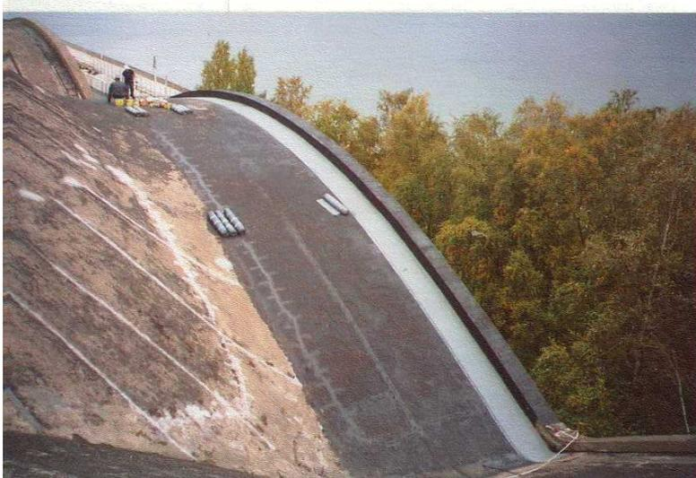
Figure 7.13 Installation of roof cover
