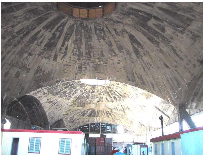
Figure 5.9 Damages of the lower surface
