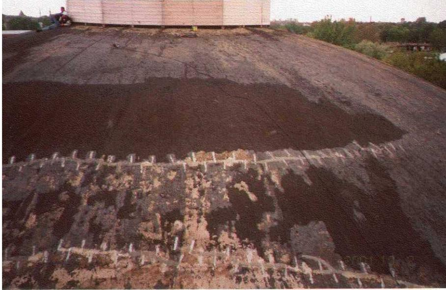
Figure 7.11 Cracks stitched and injected by epoxy resin
