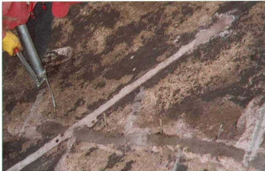
Figure 7.10 Crack injection by epoxy resin
