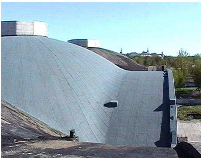
Figure 7.14 Shell coverage with SBS roof covering materials
