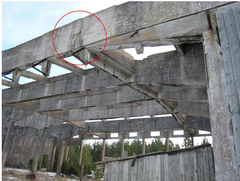
Figure 5.7 Deformation joint
