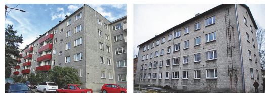
Fig. 1. Typical prefabricated reinforced concrete large-panel element apartment building (left) and brick apartment building (right)
