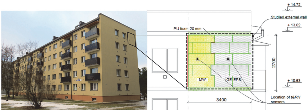
Figure 1 View to the external wall with measurement areas of ETICS.
