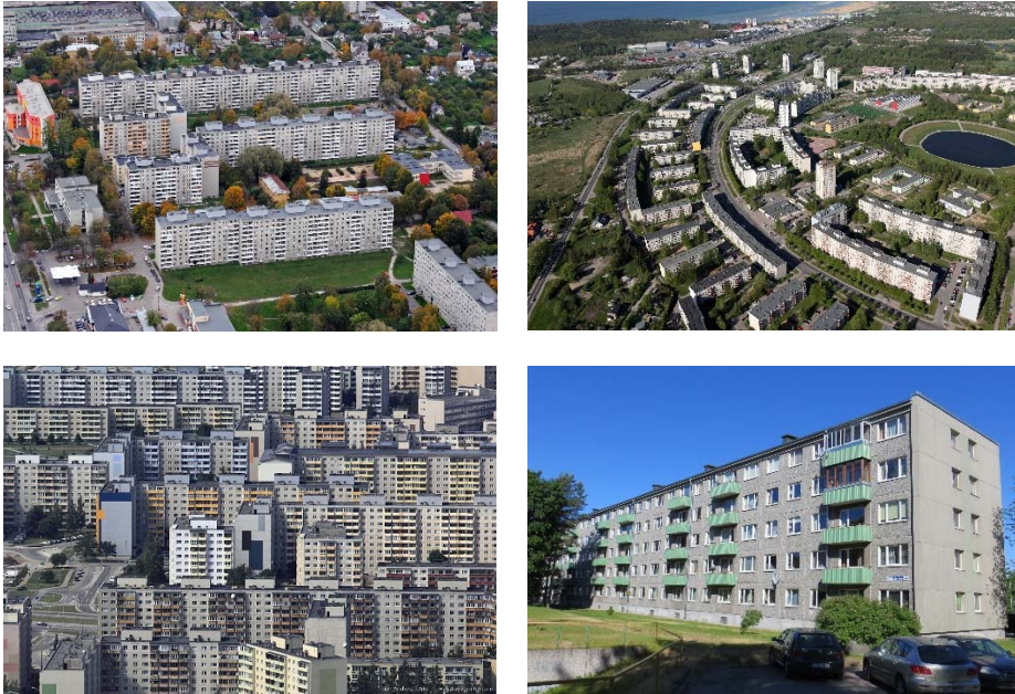
Figure 2.1. Concrete apartment buildings in districts of Tallinn – Mustamäe (top left), Õismäe (top right), Lasnamäe (bottom left), all from www.taevapiltnik.ee , and a typical 1-464 series building from Mustamäe (bottom right).
