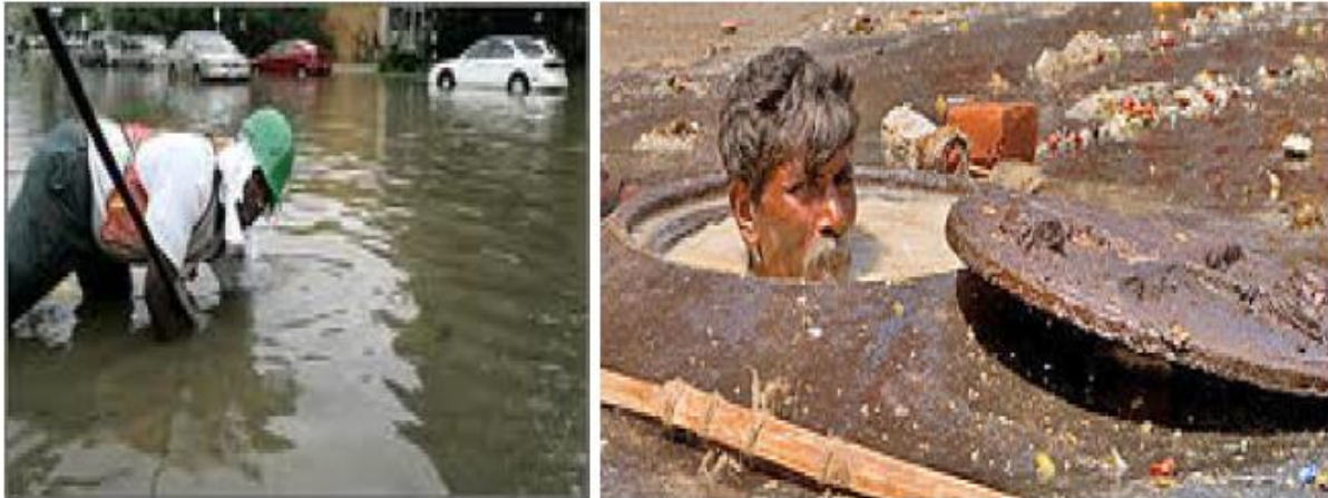
Figure 4: Troubles in pipeline failure
