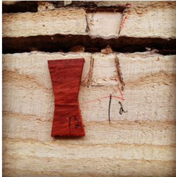
Figure 15. Bow tie(butterfly) application
