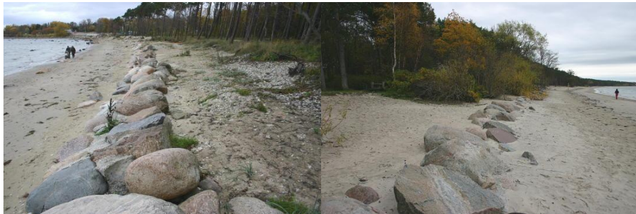
Fig. 3.3. Remnants of the revetment in the northern part of Pirita Beach
