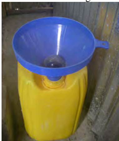
Figure 25. Eco-lilly waterless urinal in Arba Minch, small town of south Ethiopia. Source: Sustainable sanitation alliance (Sustainable sanitation alliance, 2007).
