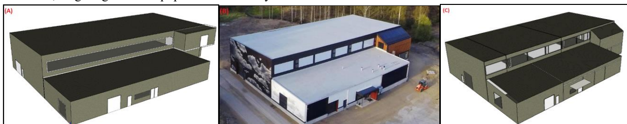
Fig. 1. (a) Initial design model in IDA ICE. (b) OLK NZEB in Hämeenlinna. (c) Building calibration model in IDA ICE
